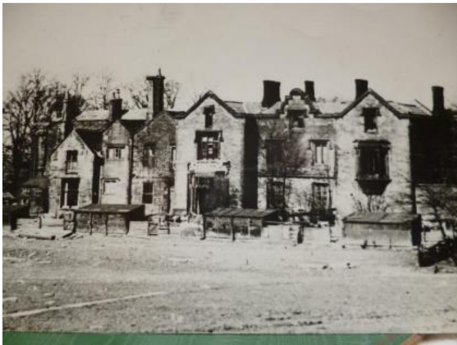
Figure 4: dilapidated south elevation, mid 20 th century (client collection)
