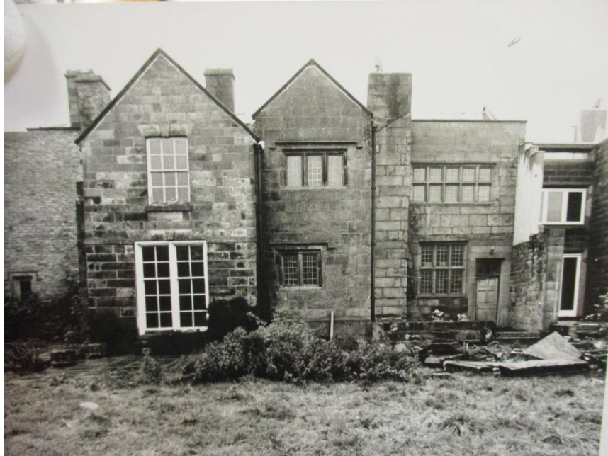
Figure 7: south elevation in c1990, before demolition of 1980s east wing (client collection)
