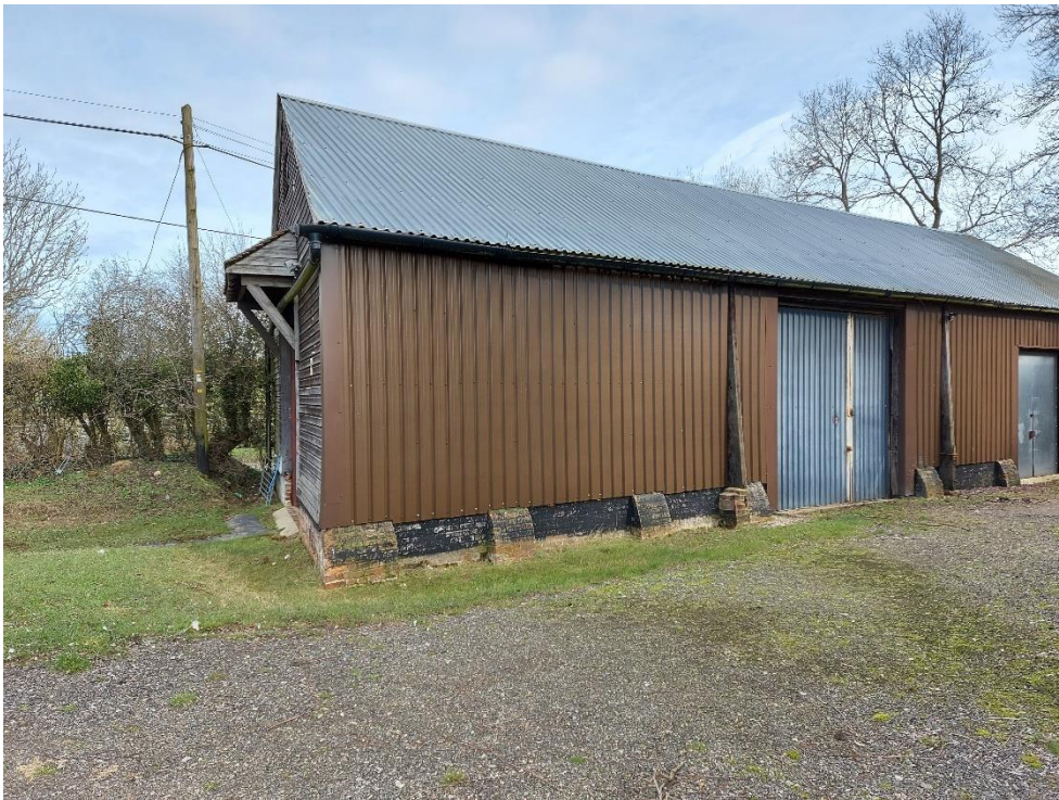
South Elevation to the rear.
