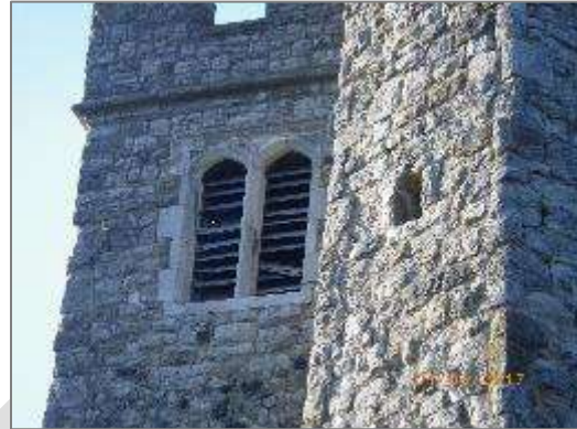
North vestry (left) and broken louvers on western tower (right)
