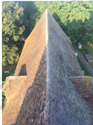
Aerial view of the nave and chancel roofs
