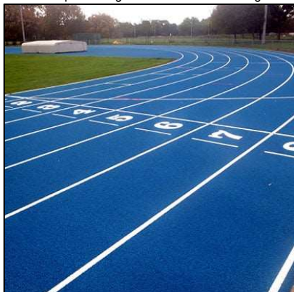
Figure 4 – sprint lane surfacing
