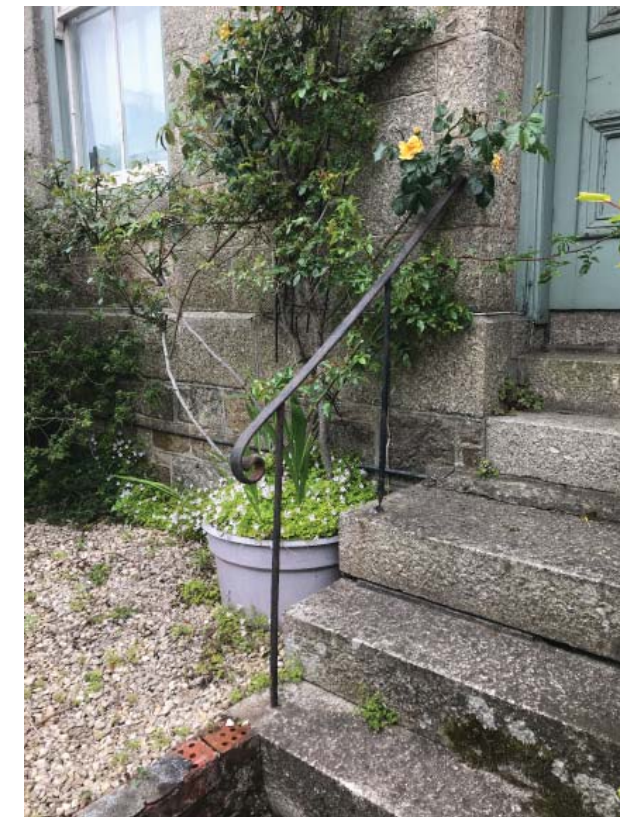
Typical Newlyn handrails and balusters
