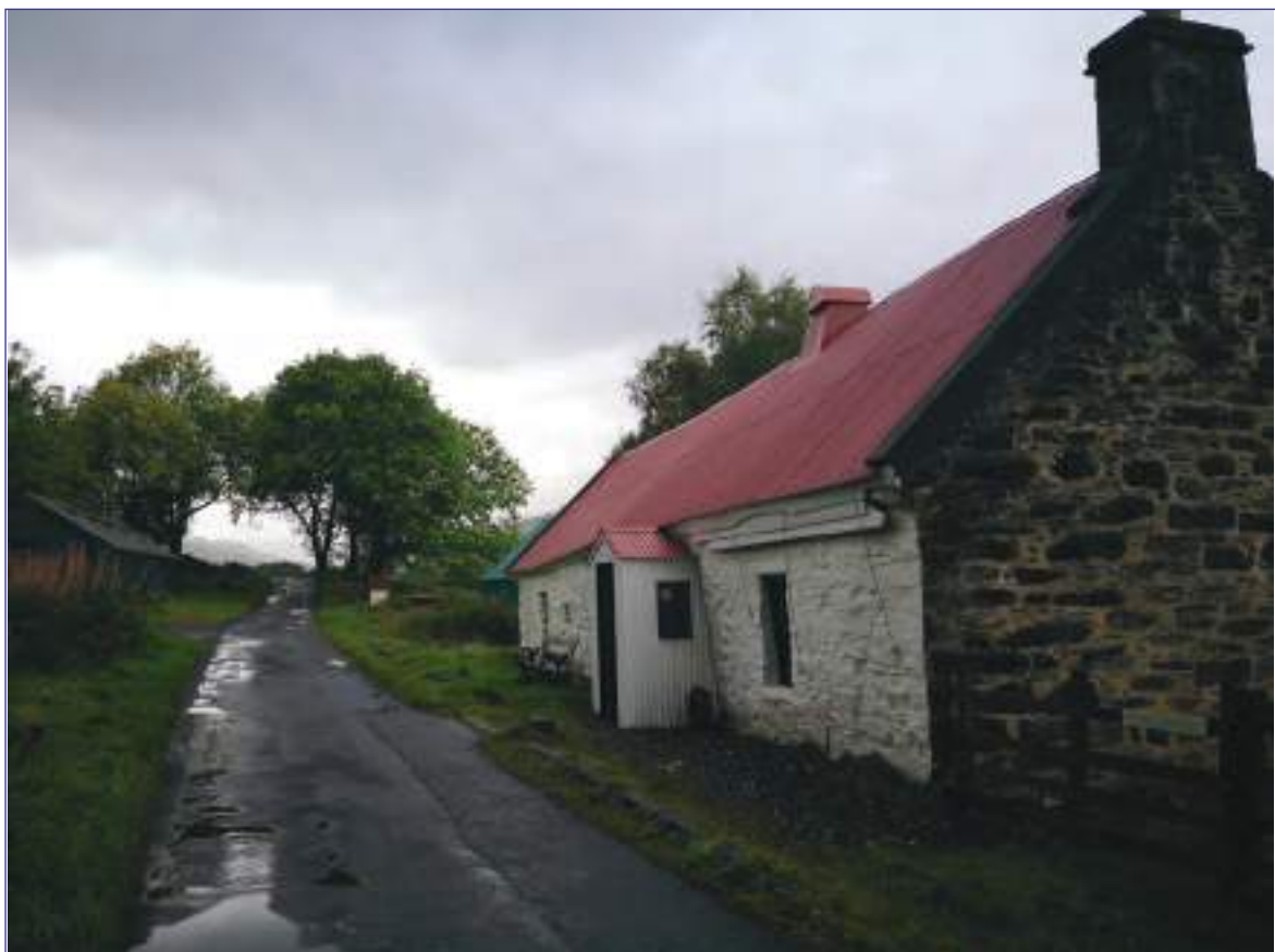
Plate 12: West facing view of the Category A Listed Moirlanich Longhouse (Site 7)
