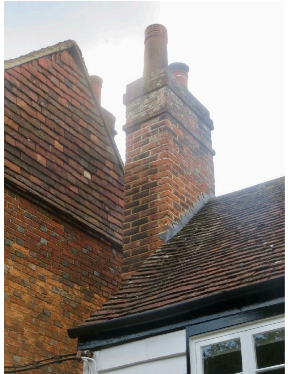
Plate 5: Upper parts of chimney and lead flashings
