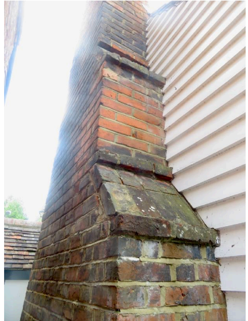
Plate 4: front elevation brick gathers
