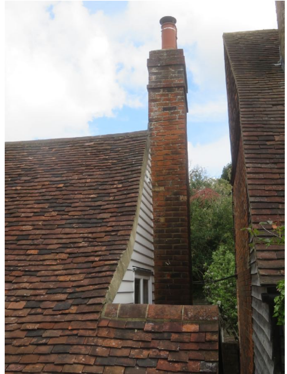
Plate 2: rear view of chimney stack
