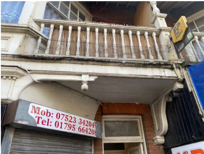
Plates 6 - The new illuminated signage will be hung within the bay soffit, concealing fixtures & fittings whilst allowing the important joinery details to be seen.
