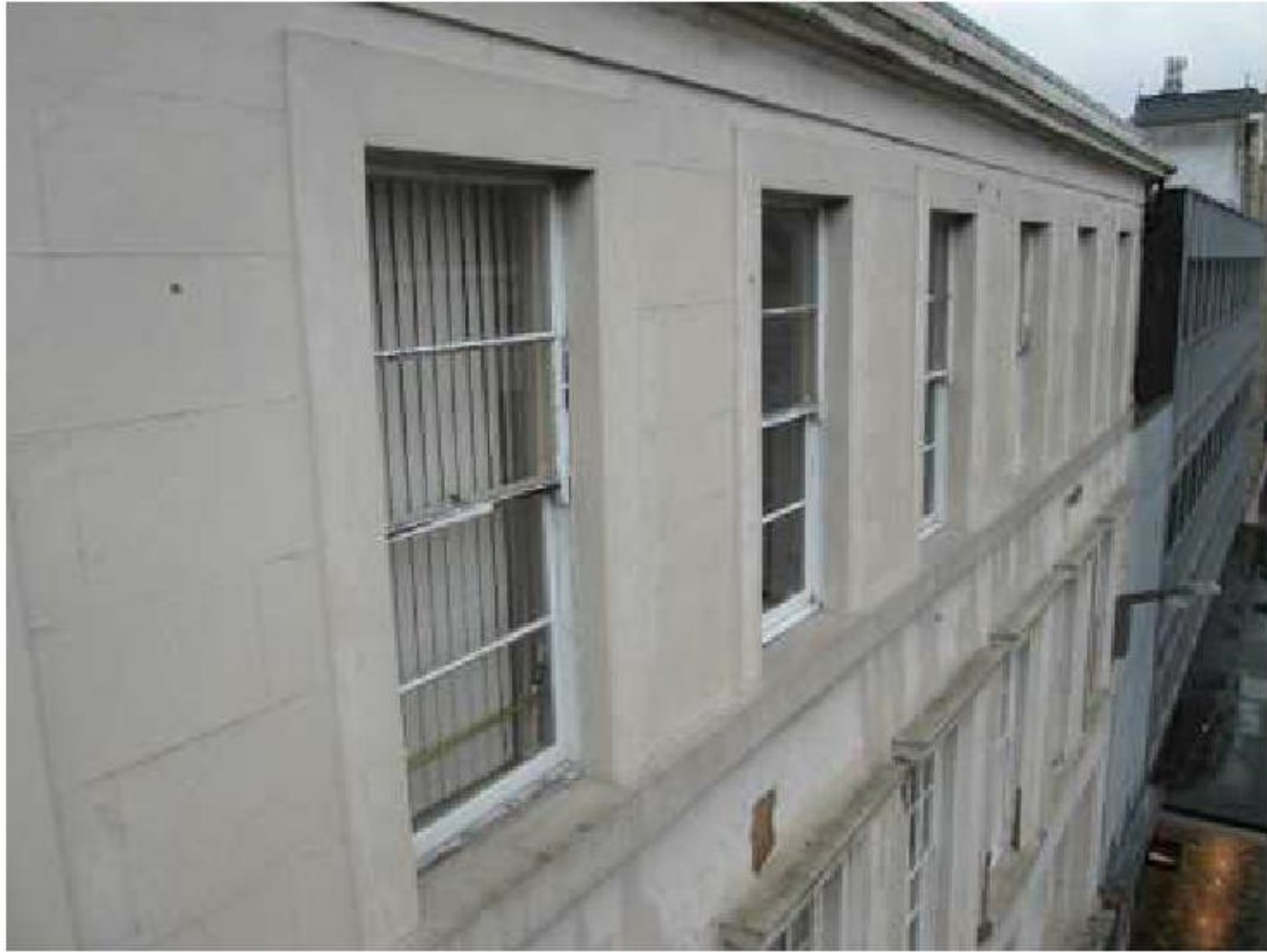
High Level Cement Render Repairs
