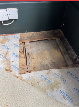
2ND FLOOR Concrete slab 50 mm to FFL
