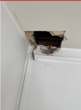
3RD FLOOR Steel beam
