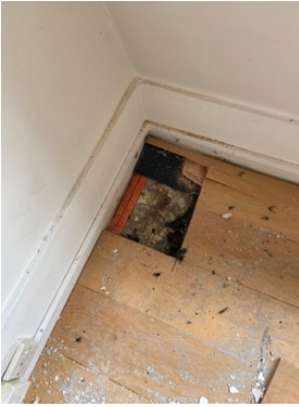
3RD FLOOR Concrete slab 40 mm to FFL
