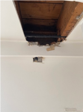
3RD FLOOR Steel beam, modern plasterboard ceiling on timber joists
