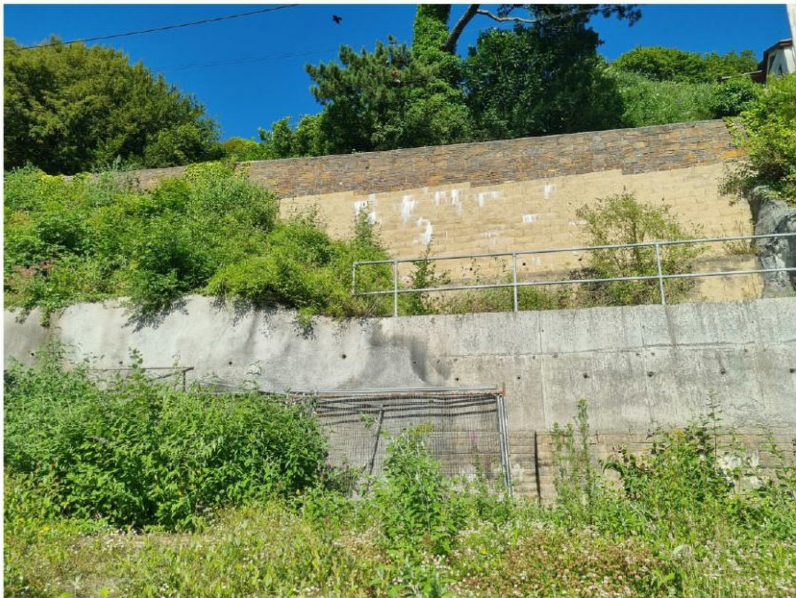
Figure 2 - Highway retaining walls to rear of site.x
