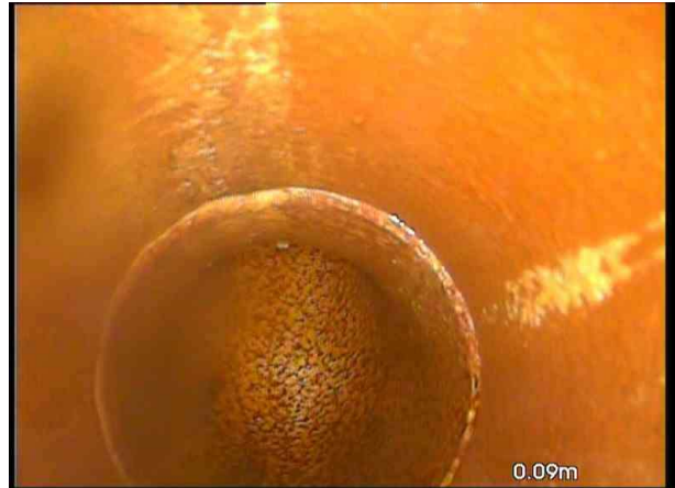
R_EX_411f8351-be1d-440f-8bb5-4e2ef0718ce6_20210831_1 13429_403.jpg, 00:00:27, 0.09 m Material changes to vitrified clay, Rest Bend
