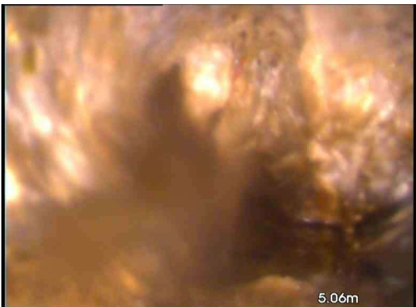
R_EX_0e705ff3-9f63-4a13-94cc-87d18df7d036_20210831_113846_055.jpg, 00:02:21, 5.06 m Roots, mass, 75% cross-sectional area loss
