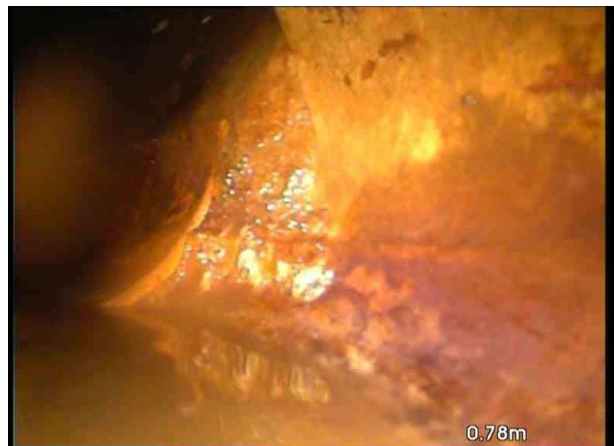
R_EX_0fbfca10-2847-4e03-bc53-ae3ceaf1fe58_20210831_11 3545_414.jpg, 00:00:44, 0.78 m Line deviates left
