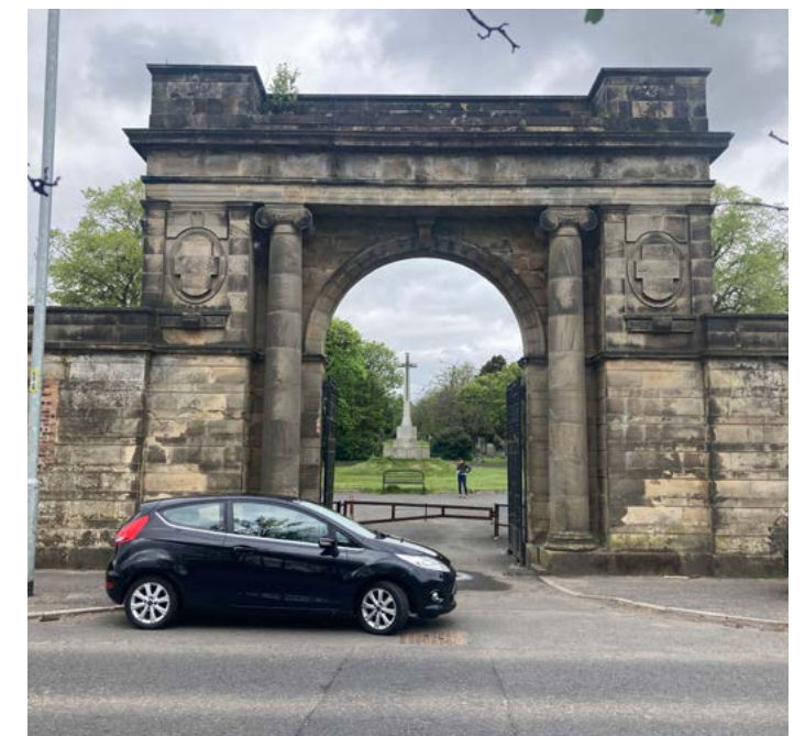
Figure 4.5 Lambhill Cemetery Entrance Arch
