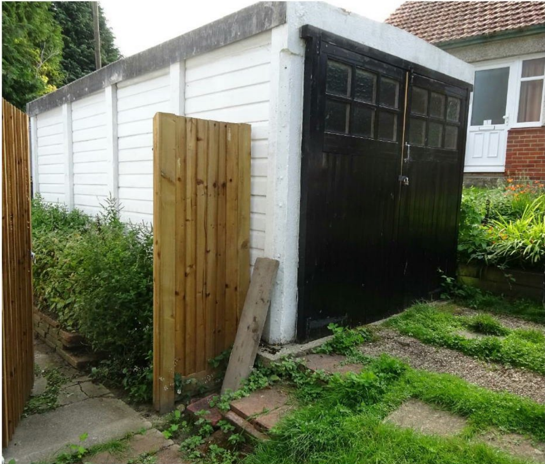
3. Existing white painted pre-fab concrete garage
