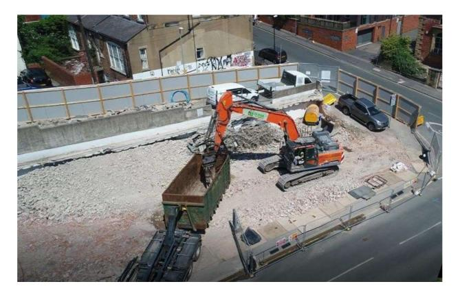
During the demolition works either a self-contained pressure washer or a standpipe and hoses will be utilised for dust suppression. The pressure washer / standpipe will be positioned outside of the immediate demolition zone. Water will be delivered into the area using the gun attachment on the bowser / hoses.
