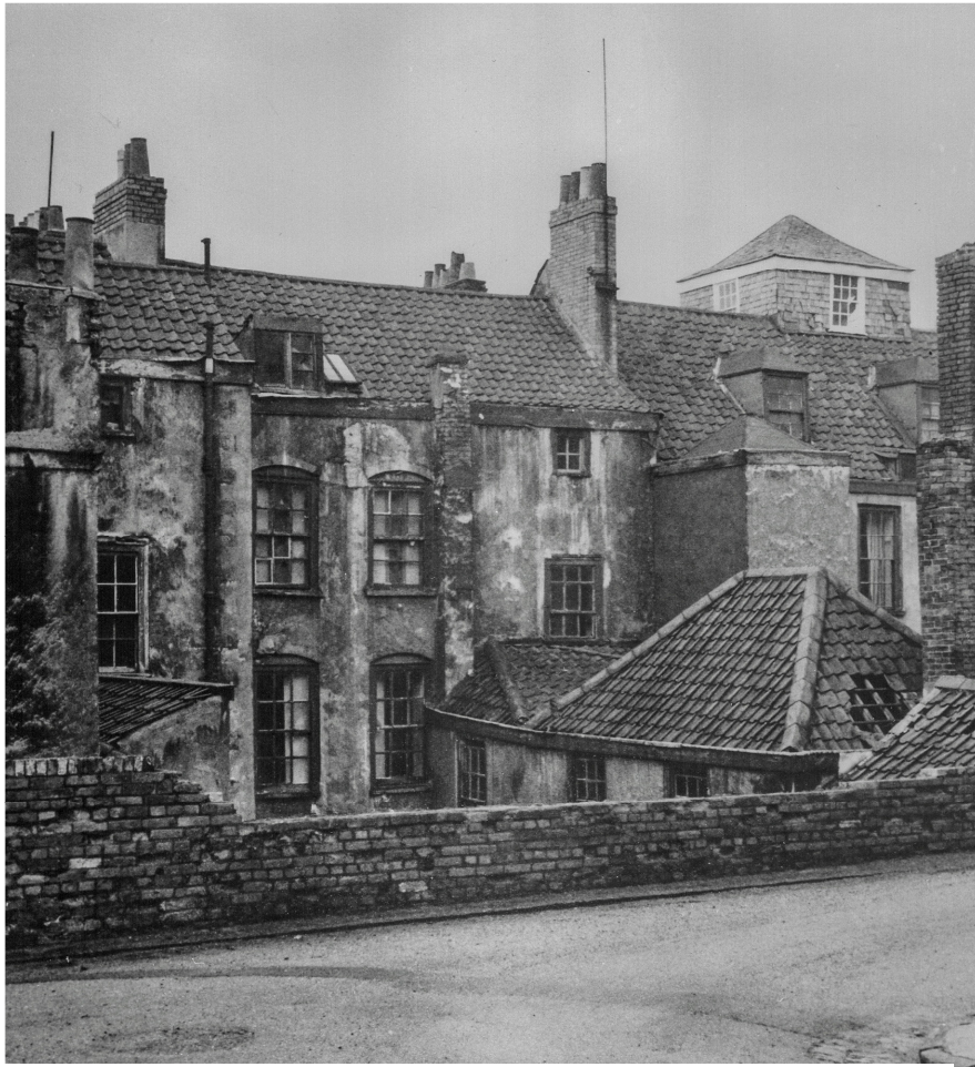
Fig. 7: View from the North (rear) elevation of No.10 Dowry Square
