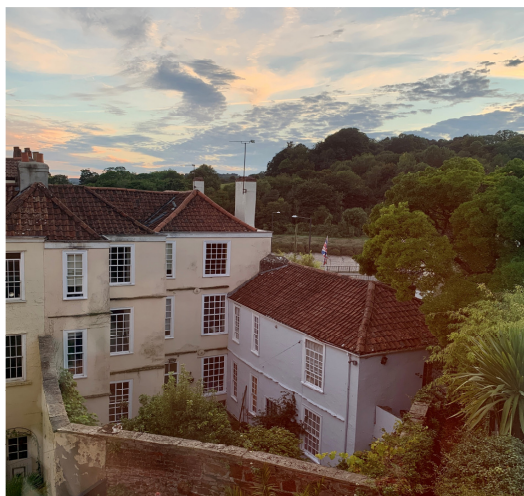
Fig.16 Historic precedent exists for two storey rear extensions to most of the dwellings along the north side of Dowry Square and in the surrounding area.
