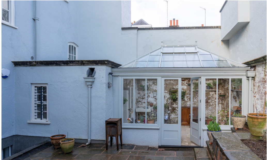
Fig.13. Existing rear extensions
