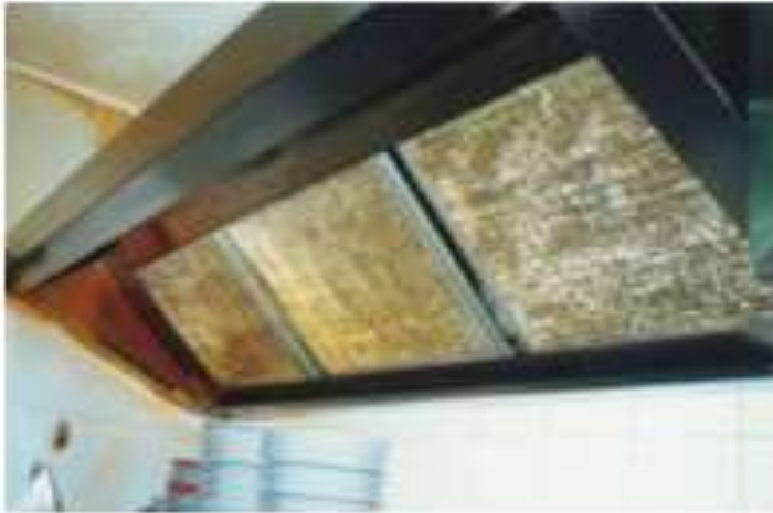
Figure 9: Example of a mesh filter [no longer recommended for primary grease separation].
