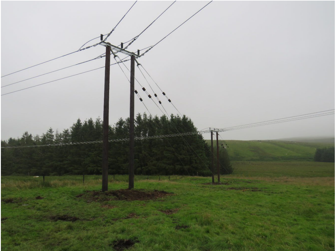
Photo 4.4: Typical Angle Pole
