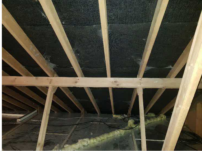
Internal loft space.
