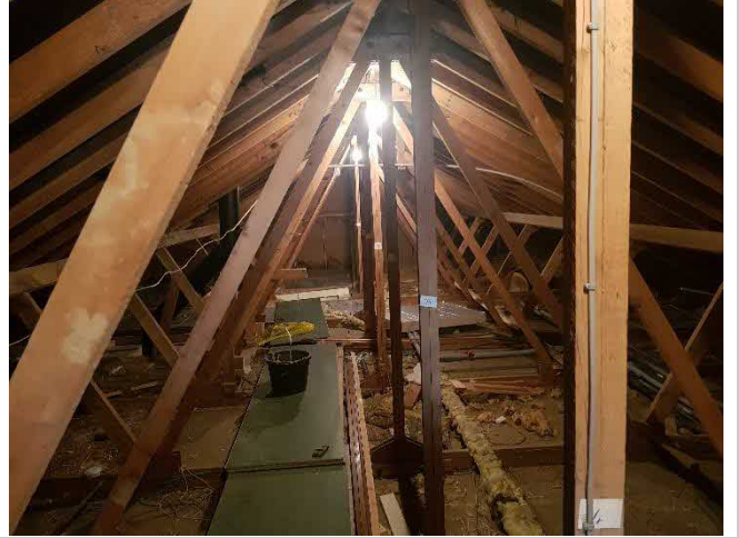
Internal loft space.
