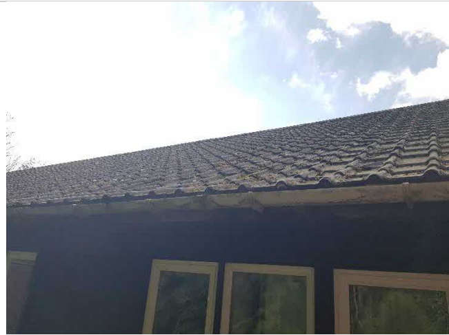
Roof at north elevation.
