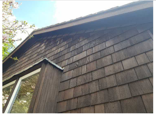
Eaves and shingle detail.
