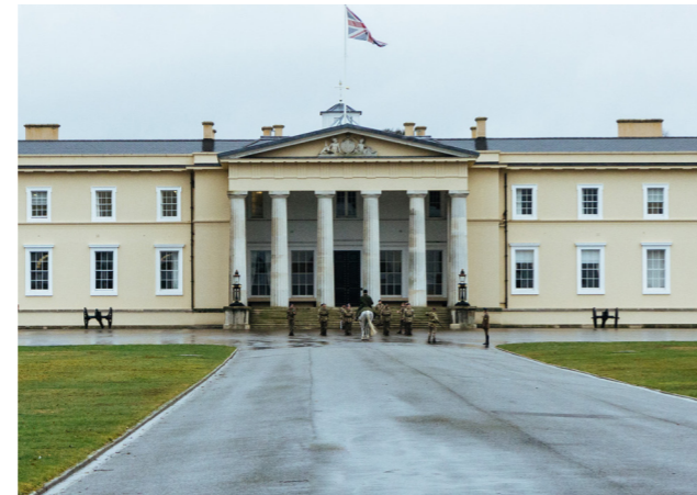
Old College - South East of Sites Source: HLM Architects
