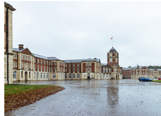
New College - South East of Sites Source: HLM Architects
