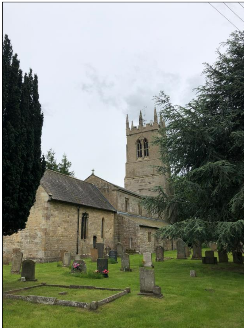
Plate 32. Grade I Listed Building NHLE 1045559 Church of Holy Trinity
