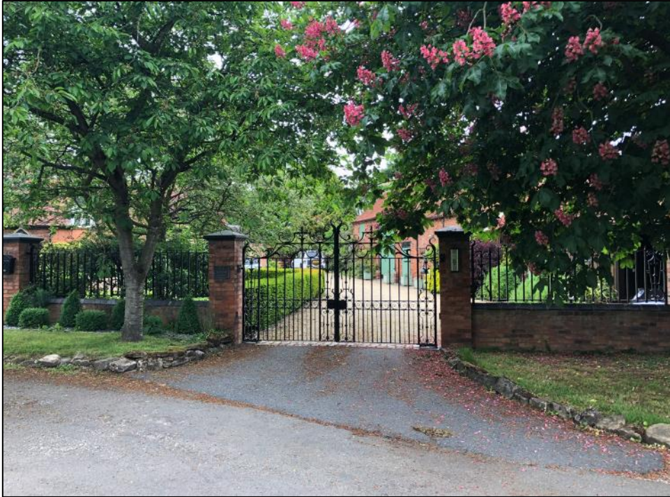
Plate 16. The front of NHLE 1370184 The Manor House
