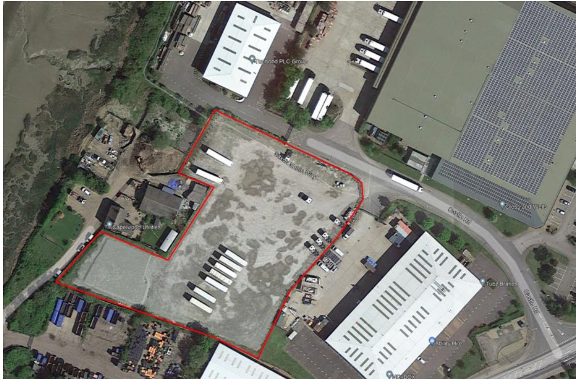
Figure 5.1: Aerial image of the site showing HGVs parked on the site dated May 2018 (courtesy of Google Earth).
