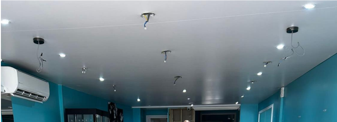
Picture 3: Ceiling and Lights.
