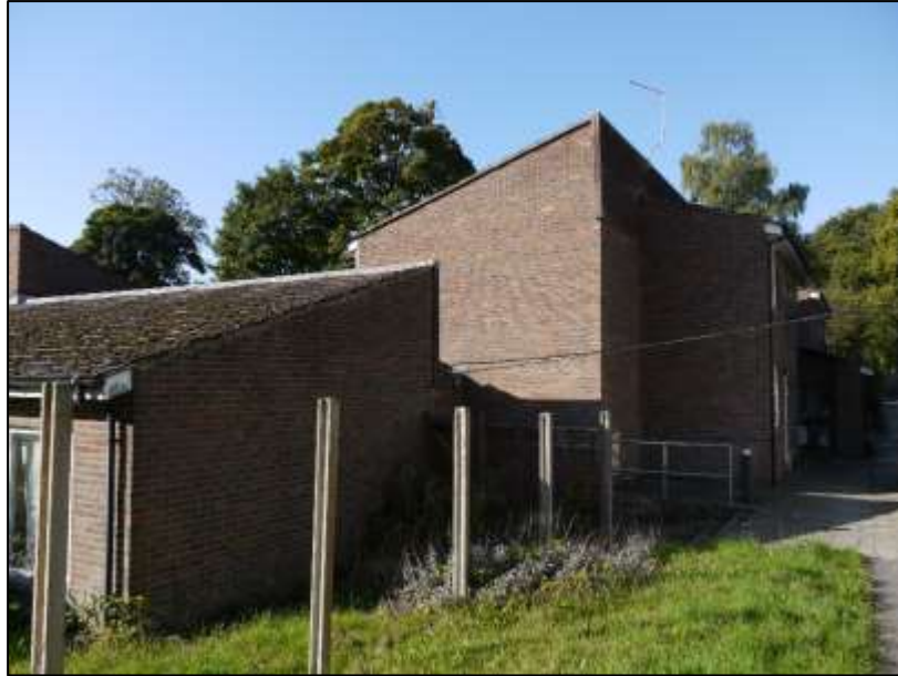
Photo 3: Northern and eastern elevation of B3.
