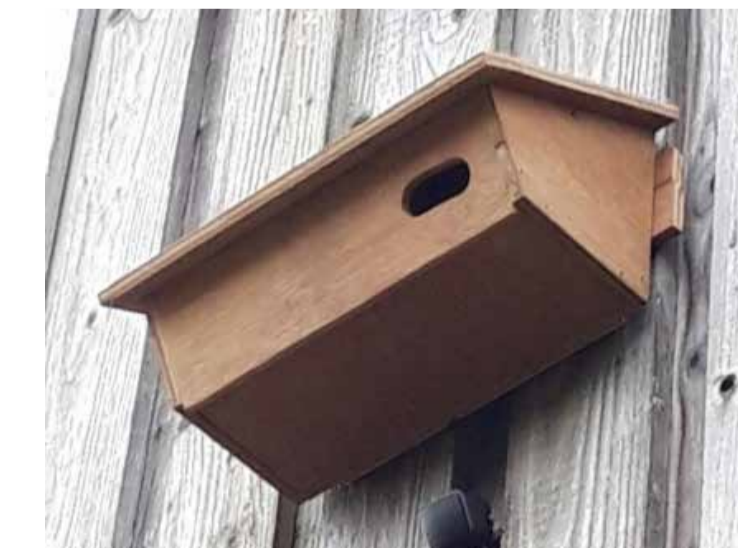
11. Provision dedicated swift boxes located on the west side of the new building.
