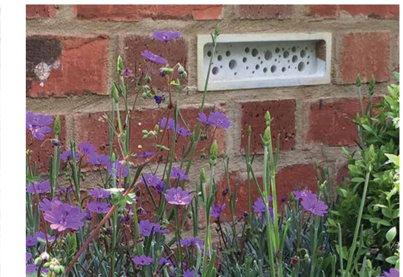
12. Proposed provision and installation of bee bricks within the masonry of the proposed new dwelling.
