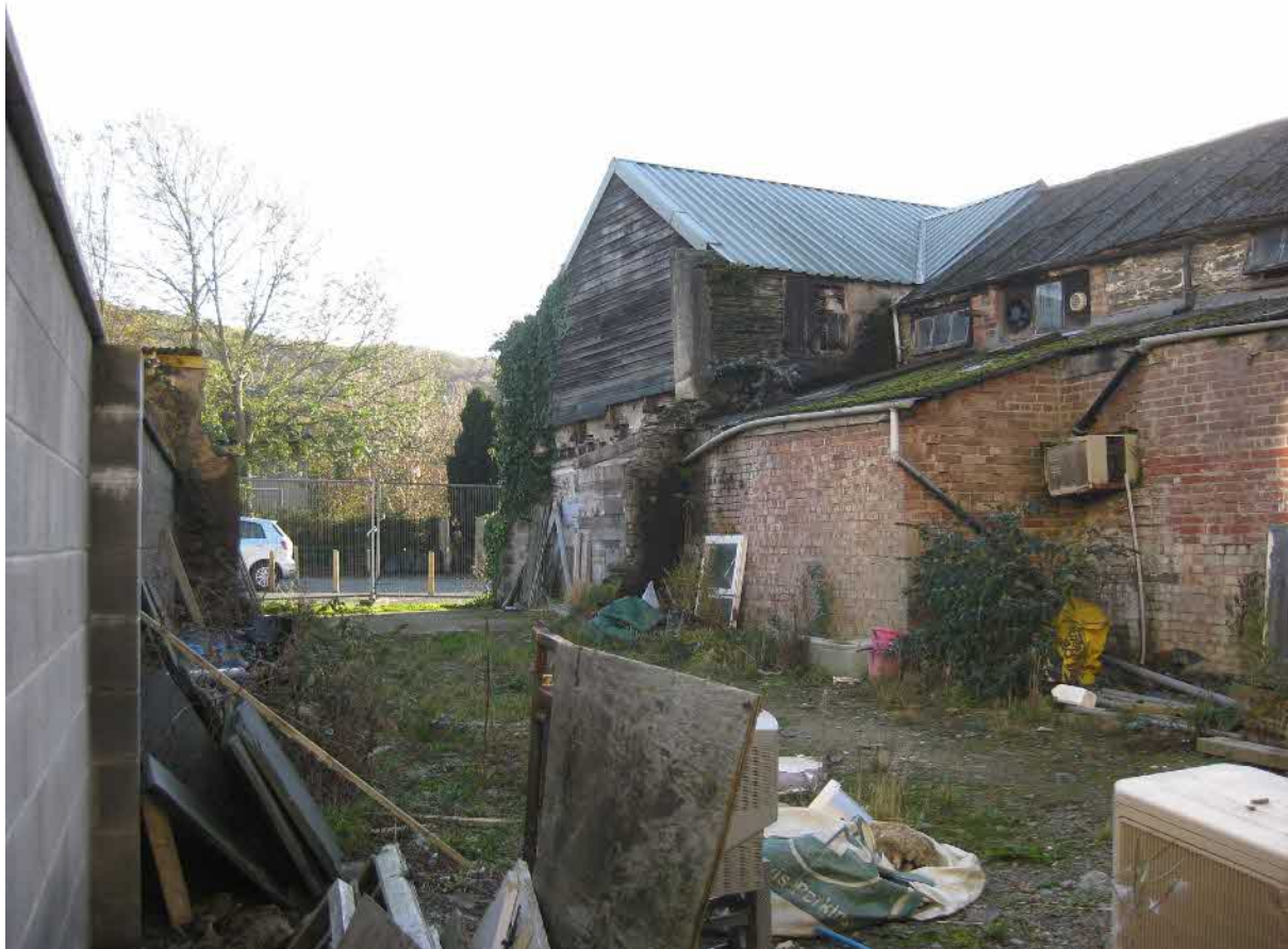
View of the southern half of the site .
