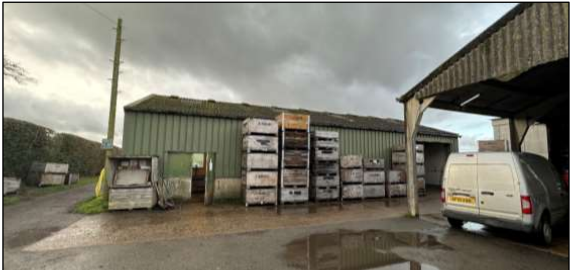
Photograph of the northern elevation of the building, taken December 2022
