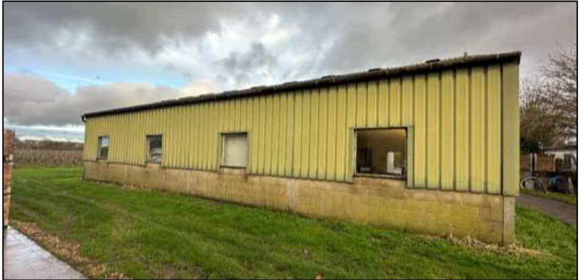
Photograph of the southern elevation of the building, taken December 2022
