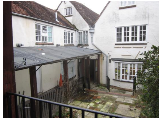
3. The internal courtyard with the covered walkway to the left.
