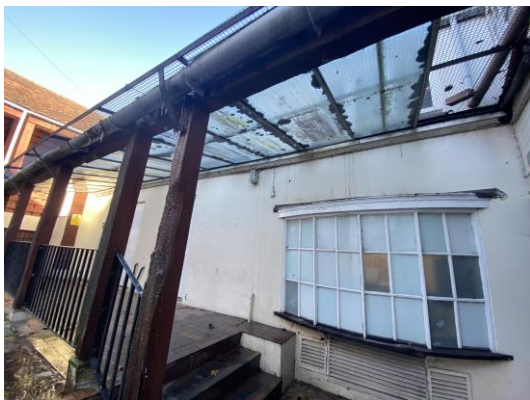
4. The walkway with the covering supported on timber posts, with railings between.
