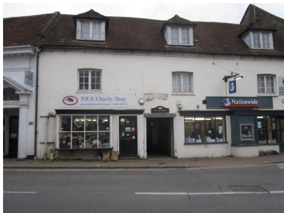
1. 2-4 High Street with the covered walkway between the two shops.
