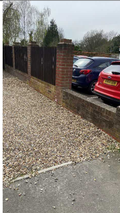
Brick wall and piers to driveway
